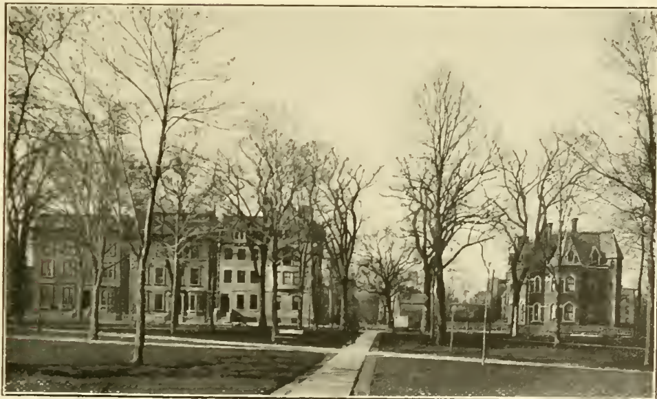
VIEW AT WASHINGTON PARK, ADJOINING WASHINGTON PLACE
